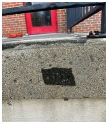
Before & after power washing: black square is before.
